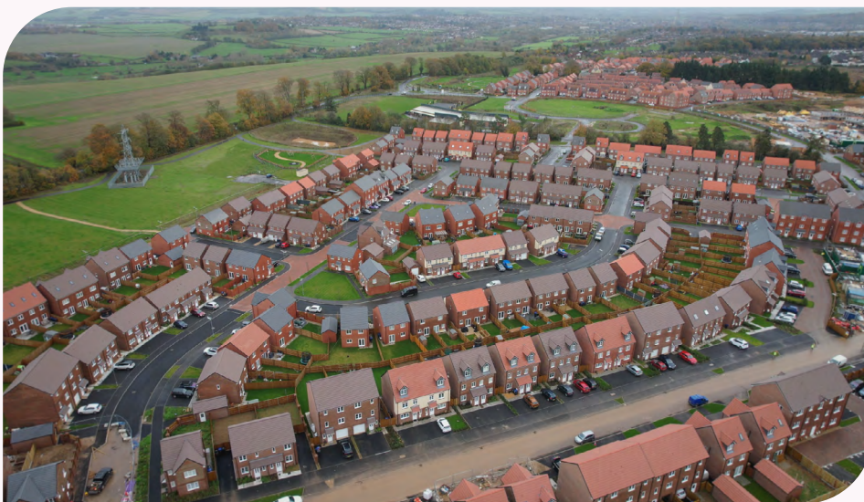
The Fugglestone development in Salisbury, which is held in the Fund's impact affordable housing portfolio
